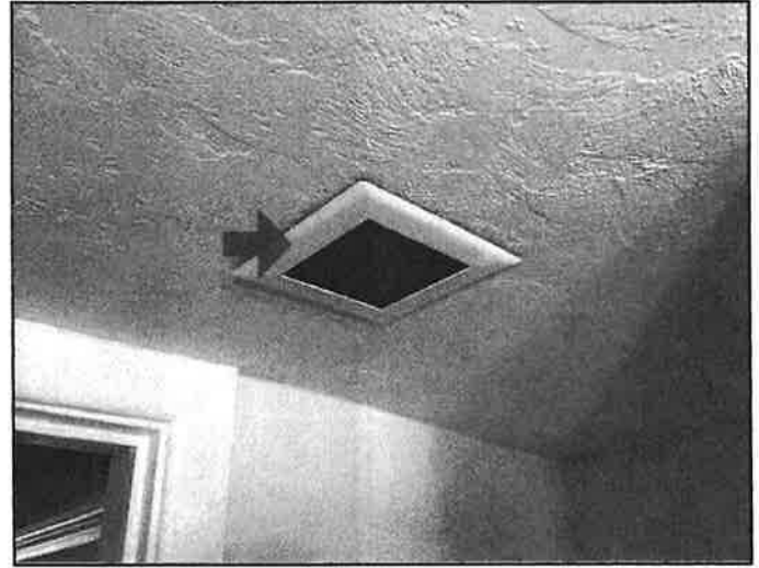
181. Second Floor Bath
