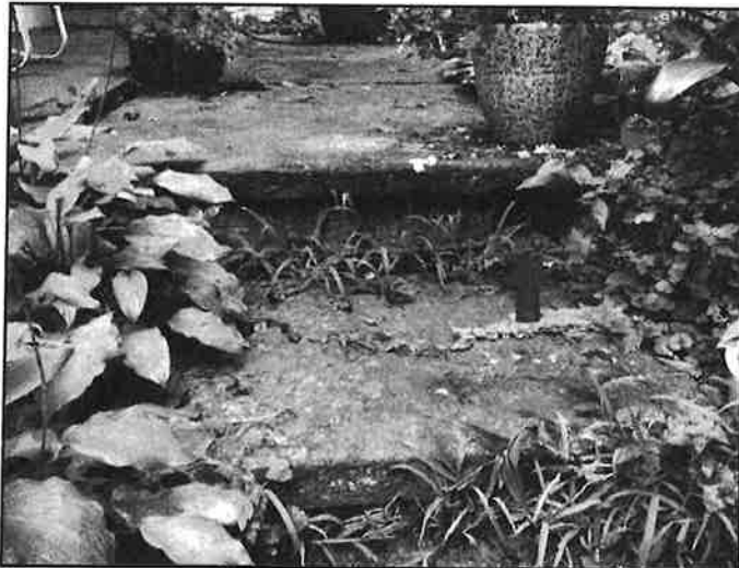
25. Missing Masonry
