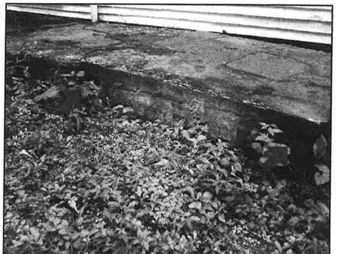
132. Deteriorated Masonry
