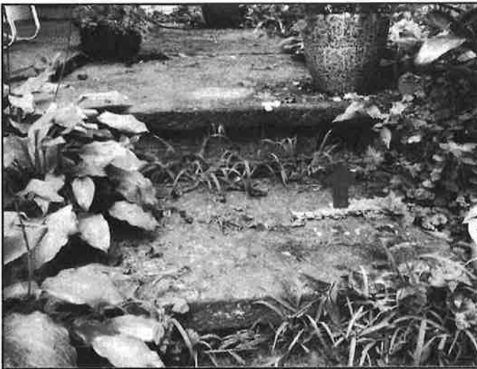
133. Missing Masonry
