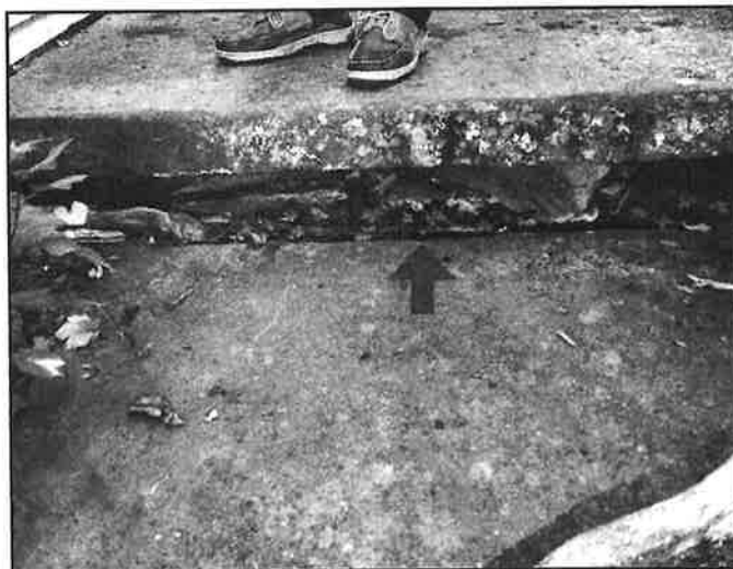
21. Deteriorated Masonry
