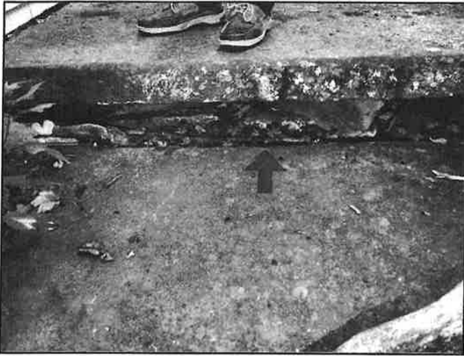
129. Deteriorated Masonry
