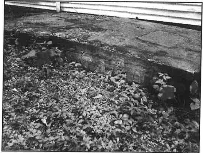
24. Deteriorated Masonry
